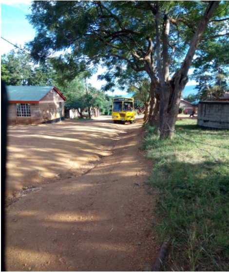
Plate 4: The deplorable school roads condition with the refurbished classroom
