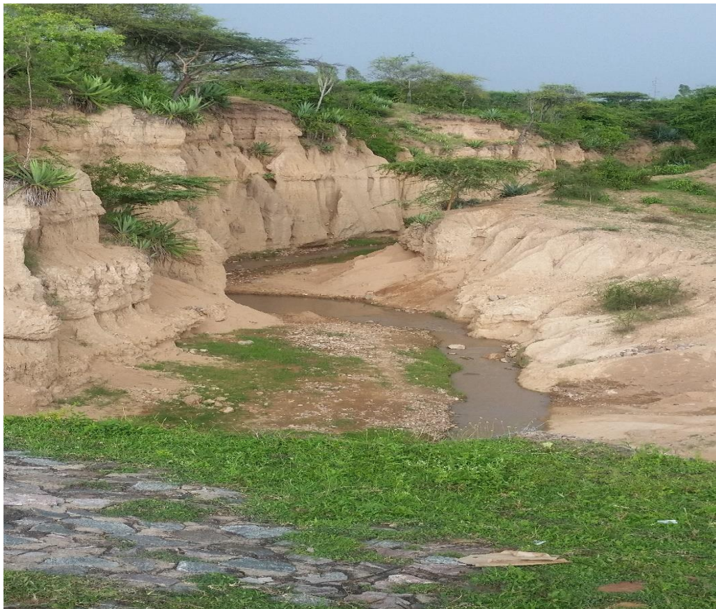
Plate 2: A Gully in an Existent Water Channel in Lower Nyakach
